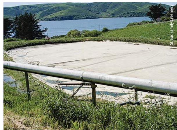
In California, dairies such as Straus Family Creamery overlooking Tomales Bay are reducing greenhouse gas emissions by converting cow manure into energy in methane digesters. Under the tarp, the liquid manure is transformed by bacteria into biogas, which powers an engine that fuels an electric generator.
