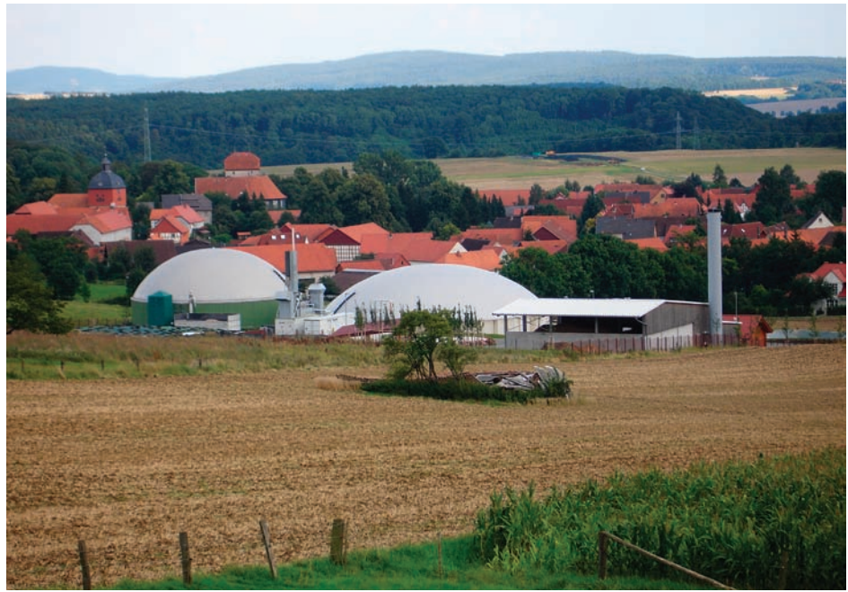
Covered lagoons and methane digesters are an option for reducing greenhouse-gas emissions from dairy waste. In Germany, the village of Juehnde built a digester for livestock waste and other biomass. The methane is combusted to produce electric power and heat for homes in the village, which is the first in the world to go “off the grid” through the use of its own waste.
