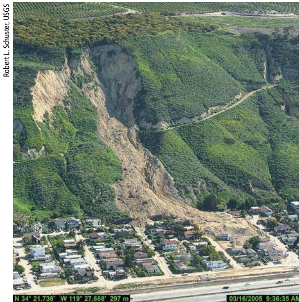
On Jan. 10, 2005, a landslide struck the community of La Conchita in Ventura County, destroying or seriously damaging 36 houses and killing 10 people.
