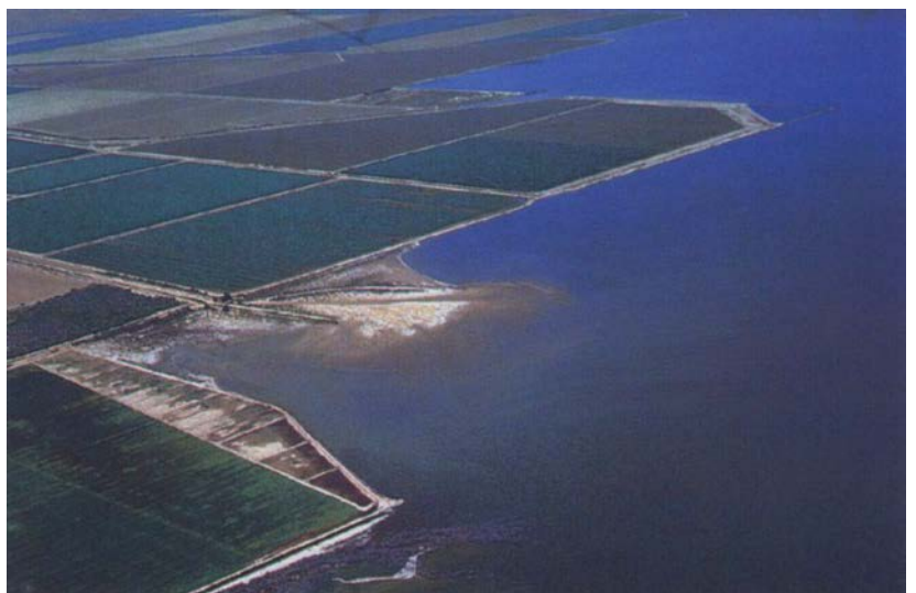
Rising water levels in the Salton Sea have flooded adjacent farmland and other property.
