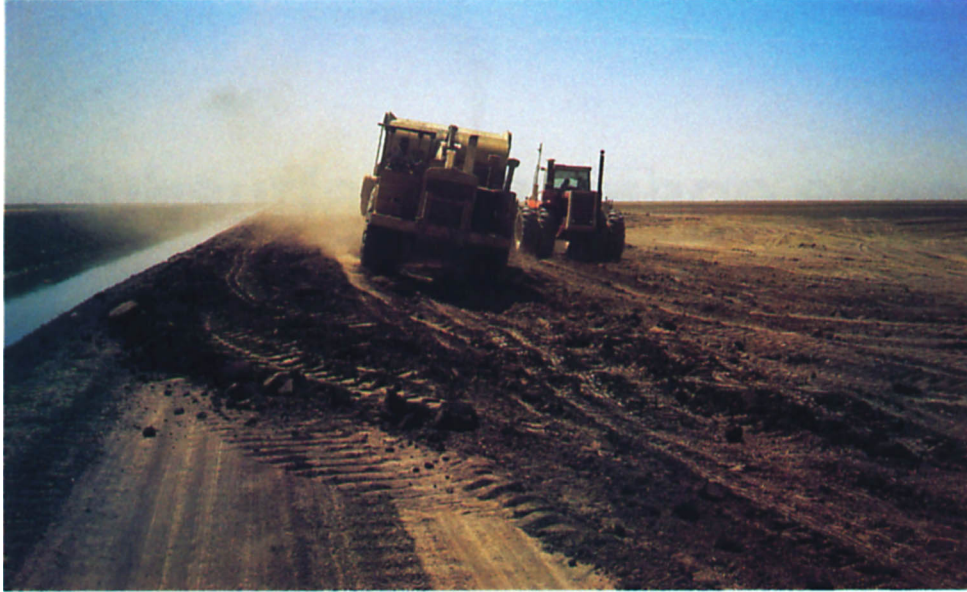
Subsurface drainage evaporation ponds, which may take more than a quarter of the land being drained out of production, have to meet rigid state standards to minimize possible adverse environmental effects. Below, drainage water is pumped from a subsurface collection system to pond surface. About 50 inches of saline water per year can be disposed of through pond evaporation. (Photos courtesy George True).
