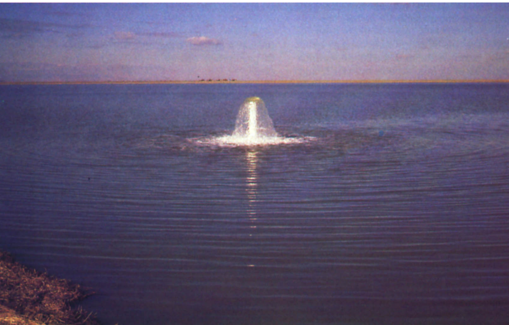
Subsurface drainage evaporation ponds, which may take more than a quarter of the land being drained out of production, have to meet rigid state standards to minimize possible adverse environmental effects. Below, drainage water is pumped from a subsurface collection system to pond surface. About 50 inches of saline water per year can be disposed of through pond evaporation. (Photos courtesy George True).
