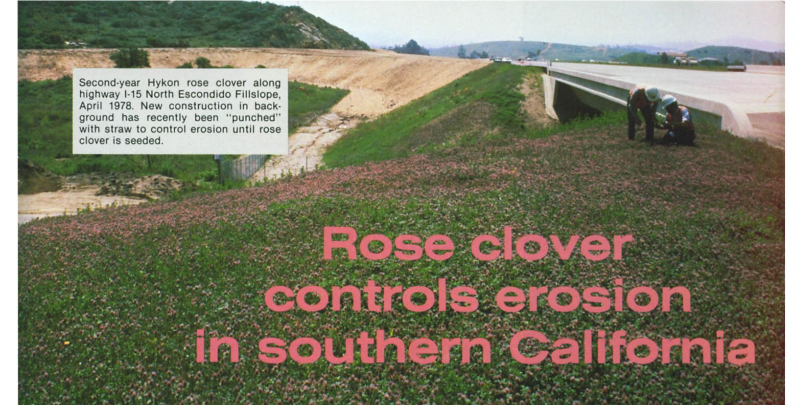
Second-year Hykon rose clover along highway I-15 North Escondido Fillslope, April 1978. New construction in background has recently been "punched" with straw to control erosion until rose clover is seeded.
