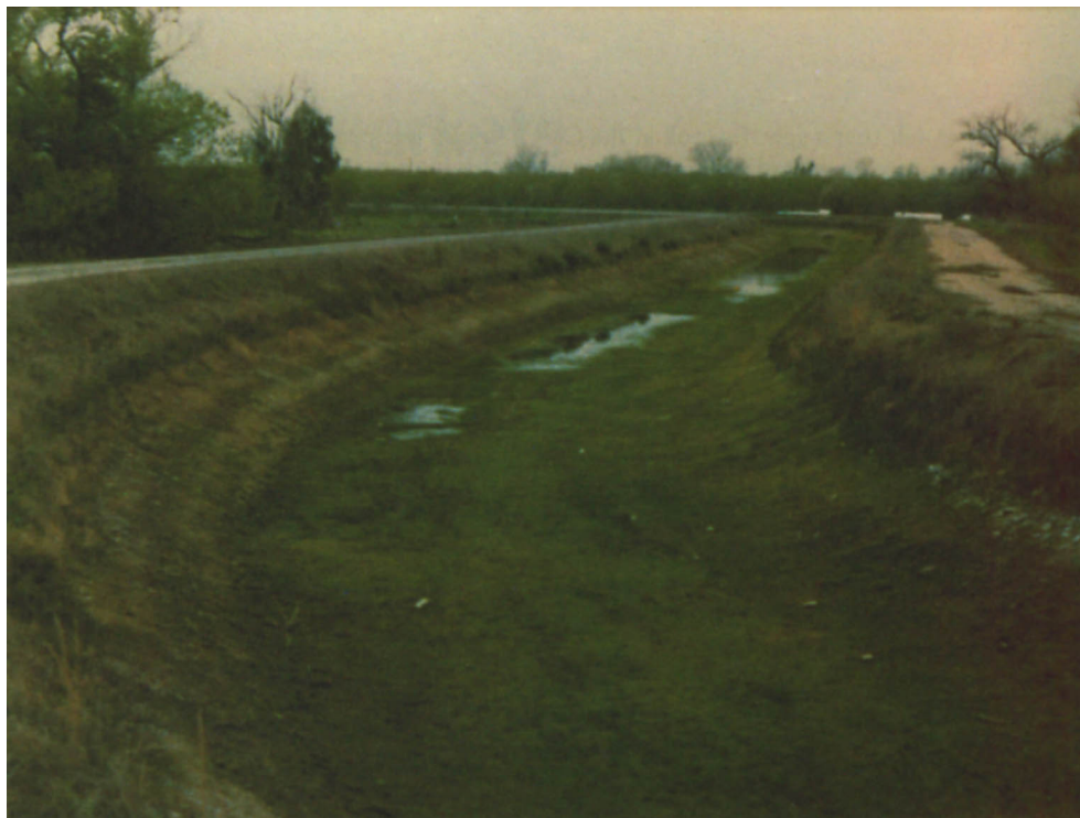
Dense sod of dwarf spikerush covering the bottom of the Corning Canal has replaced the sago, curlyleaf, and slender pondweeds that previously grew there. Water flows have increased as a result.
