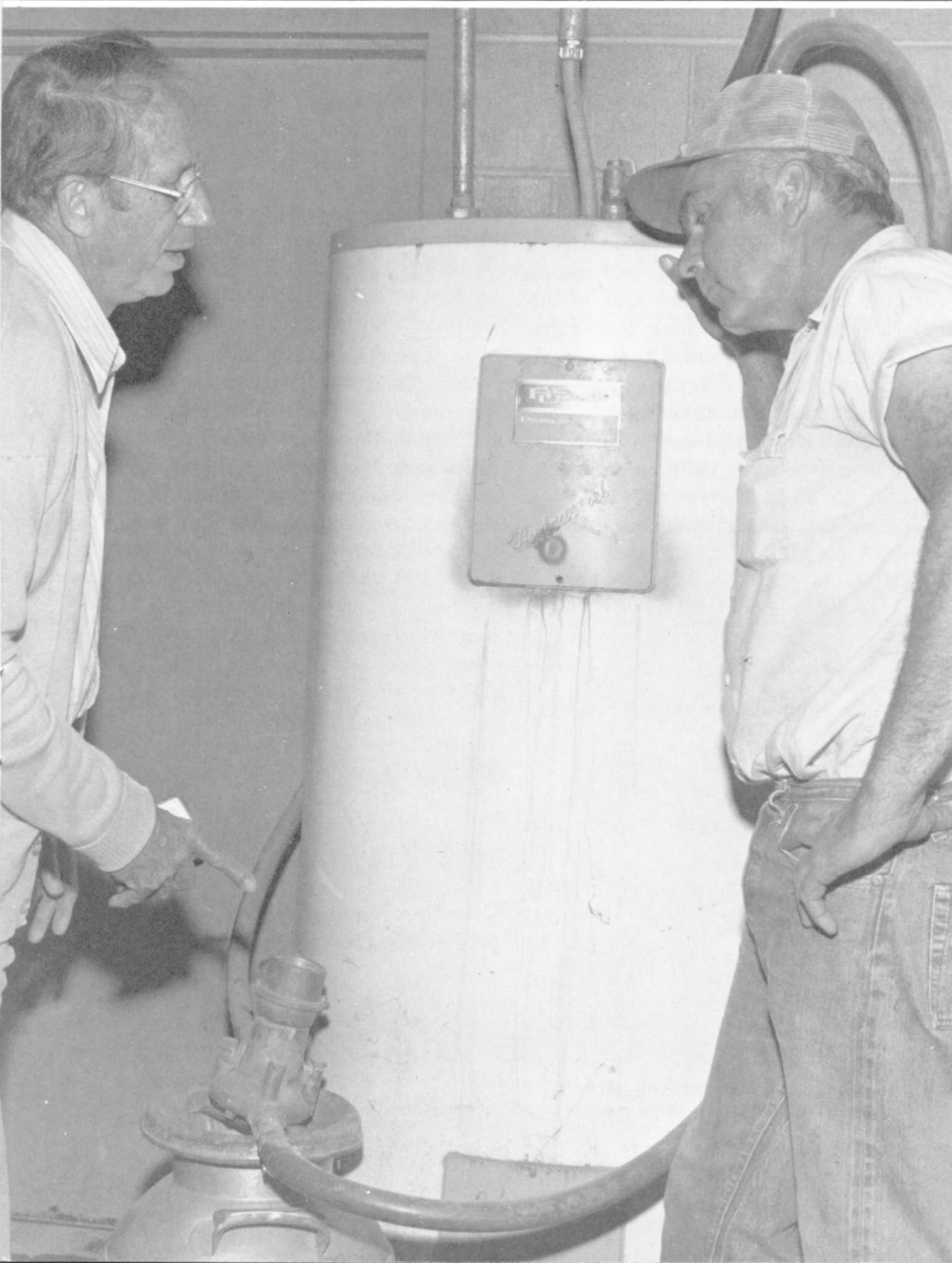
Above: Dairy Farm Advisor Richard Eide, Extension Agricultural Engineer William Fairbank, and Dairy Farm Advisor Herbert Etchegaray take note of refrigeration system head pressure to determine the limits of waste heat recovery. Below: Etchegaray reads the water meter installed by Hanford Dairyman Henry Veenendaal to record hot water usage.
