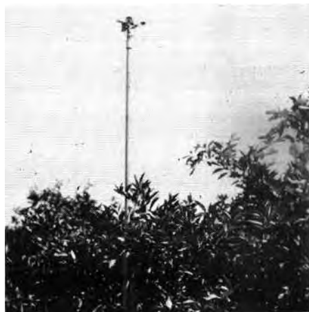
Part circle overhead sprinkler used on edge of orchard.
