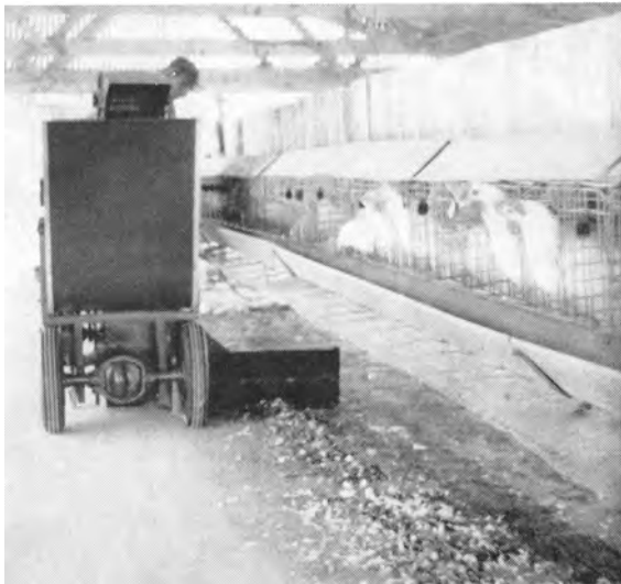
Manure cleanout machine for undercage removal of chicken manure.
