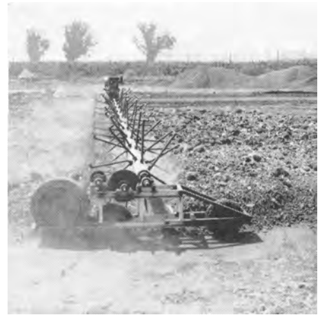
Hastened natural drying of chicken manure using a center-pivoted rotary tiller.
