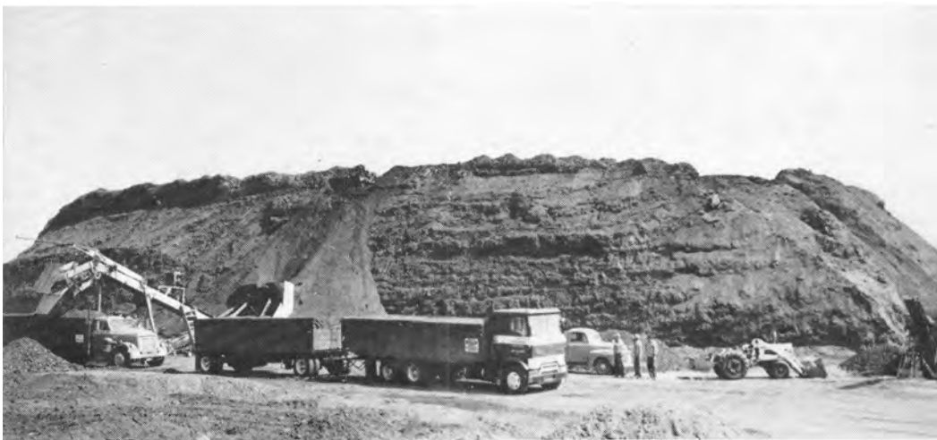
Manure stockpile of the Dairyman's Fertilizer Co-op, Inc., of Los Angeles County, California.
