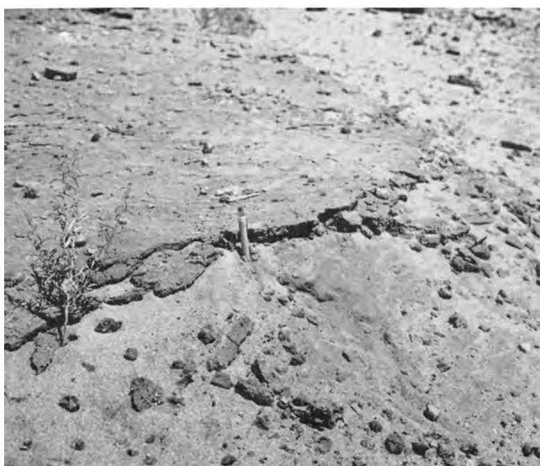
Close-up of plots 1 and 2, as located in photo on opposite page, shows undermining of the treated plot; however, the treated surface breaks off in rather large rigid blocks.
