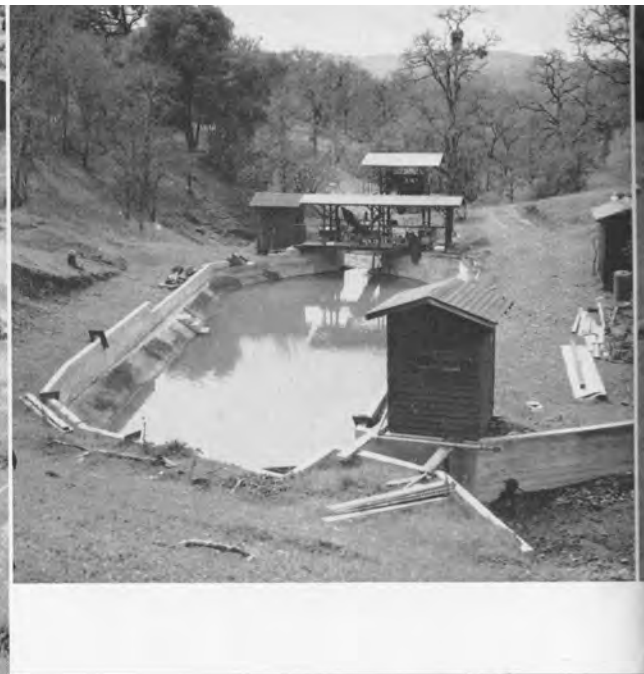
Hydrologic installation for the study of erosion and water yield in a watershed unit.
