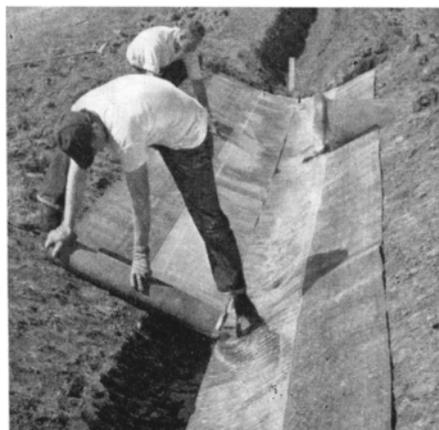
Sealing the transverse joints of the surface type lining—Asphalt C.
