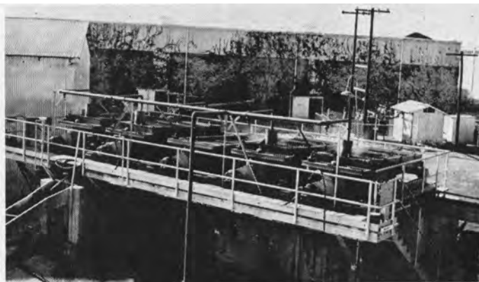
Vibrating screen solids separators for removal of pomace from stillage.
