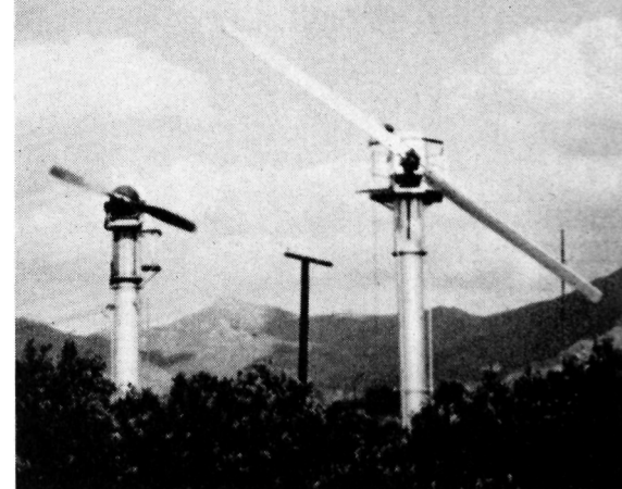
Helicopter blades on the right are 2\frac{1}{4} times as large as the standard propeller blades on the left and had a uniform turning speed 4\frac{1}{2} min./ 360^\circ , with no cold area at base of tower. The average of five tests in a 6.9^\circ F inversion show the 2^\circ F response from 200' updrift to 400' down-drift.
