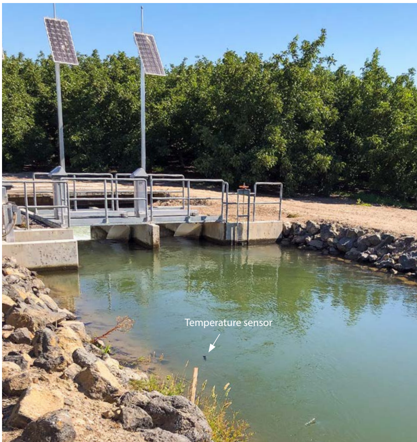
A water temperature sensor visible in the water, near an automated gate (background). Photo: AJ Borba.
