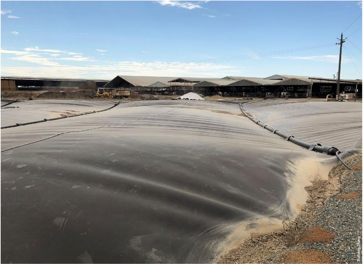
production of methane — but it recovers, or captures, the gas that would have otherwise been emitted. The captured biogas can be used to produce renewable electricity or processed to produce pipeline-quality natural gas (or renewable compressed natural gas). This energy can then be used in the operation on site or marketed to customers elsewhere.
