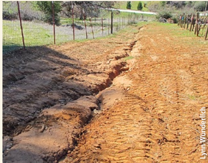
Sheet and rill erosion on an unimproved dirt road. Rills are the channel networks. Areas of sheet erosion are the smooth textured surface soil surrounding the rills.
