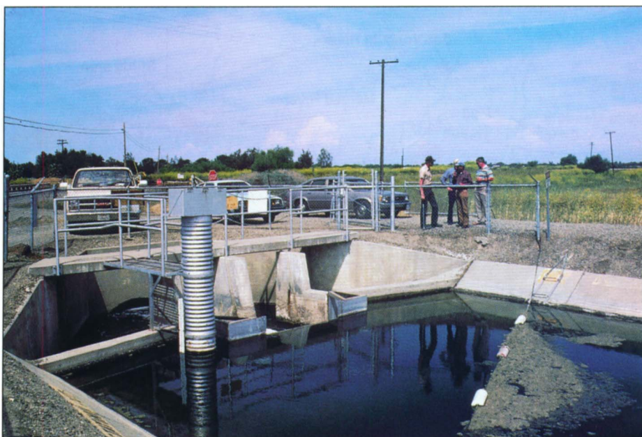
Comparisons of monthly selenium loads calculated at sites upstream and downstream allow water managers to estimate potential in-transit losses in the San Luis Drain. Flow, salinity and selenium are monitored at both sites.
