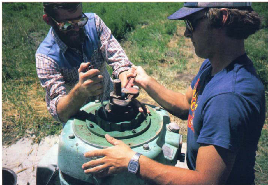
Adjustments to impellers, made by turning the nut at the top of the pump shaft, can improve pump efficiency. But that may not necessarily translate into energy savings, unless operating time is reduced.
