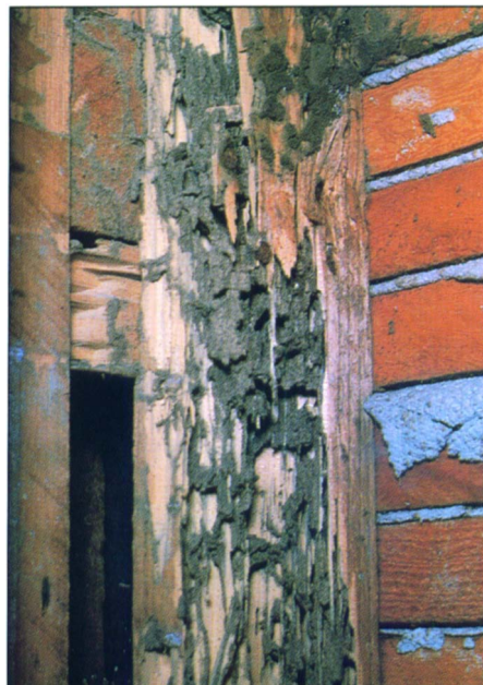
Wood damage and typical mud carton material packed in the wood by Formosan subterranean termites.
