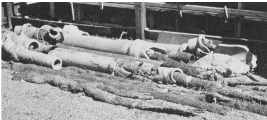
Examples of tree roots plugging sewer lines in Sacramento County.
