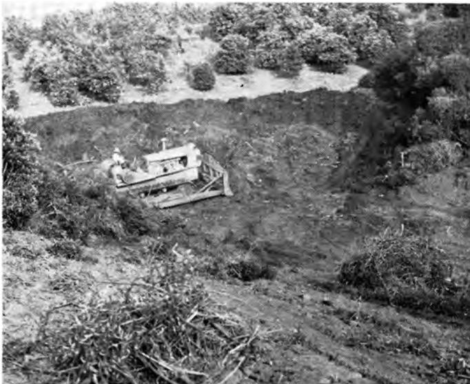
Grass seeding on steep slope at the test site was done with a range-land drill pulled by a crawler tractor.
