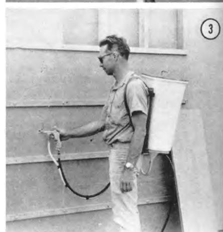
Equipment and technique used in "built-in" pest control during construction of a building: (1) "Blasto" applicator of silica aerogel dust (Dri-Die 67) as it comes from the factory; (2) applying dust in a void below the fire board; (4) dead (from desiccation) Oriental cockroach.
