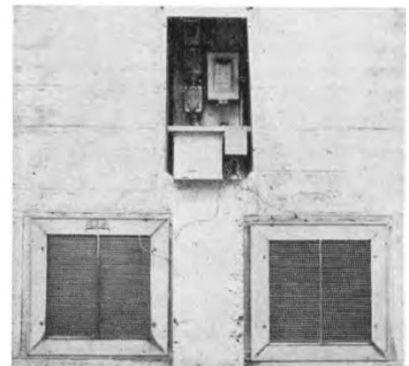
Modified form of "Champion Fly-Insect Electro-cutor" installed in the vent openings.
